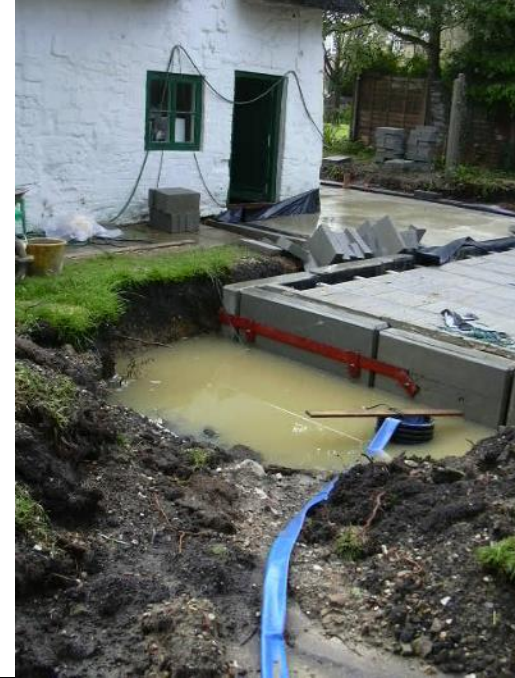
Pumping out site
