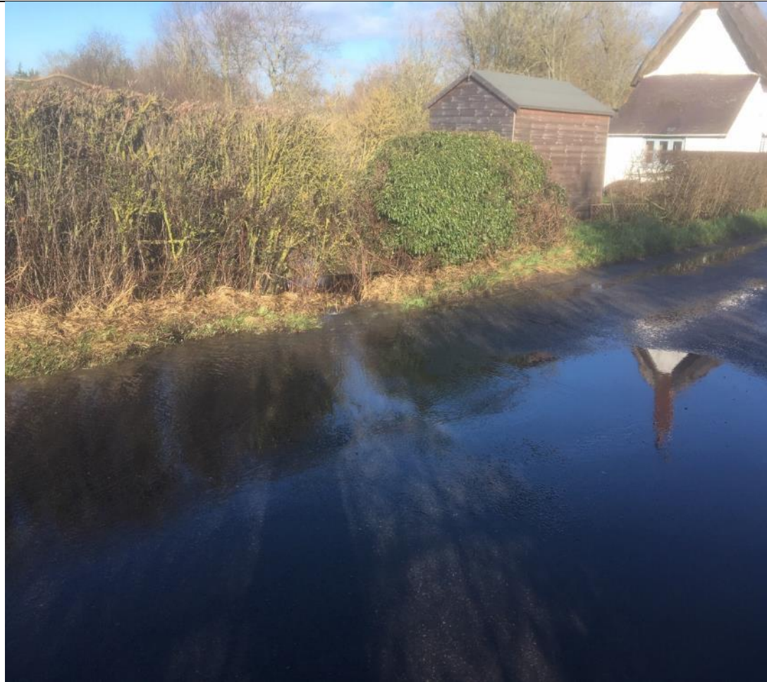
Woolstone Road outside Bridge Cottage – Jan 20
