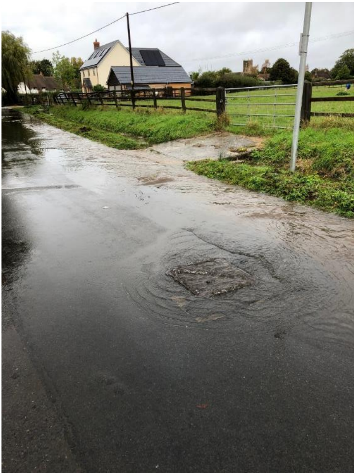
Woolstone Road/Shotover Corner – Nov 23 – note sewer bubbles from hydraulic flooding
