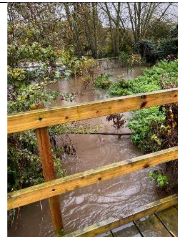
Allotments footpath bridge
