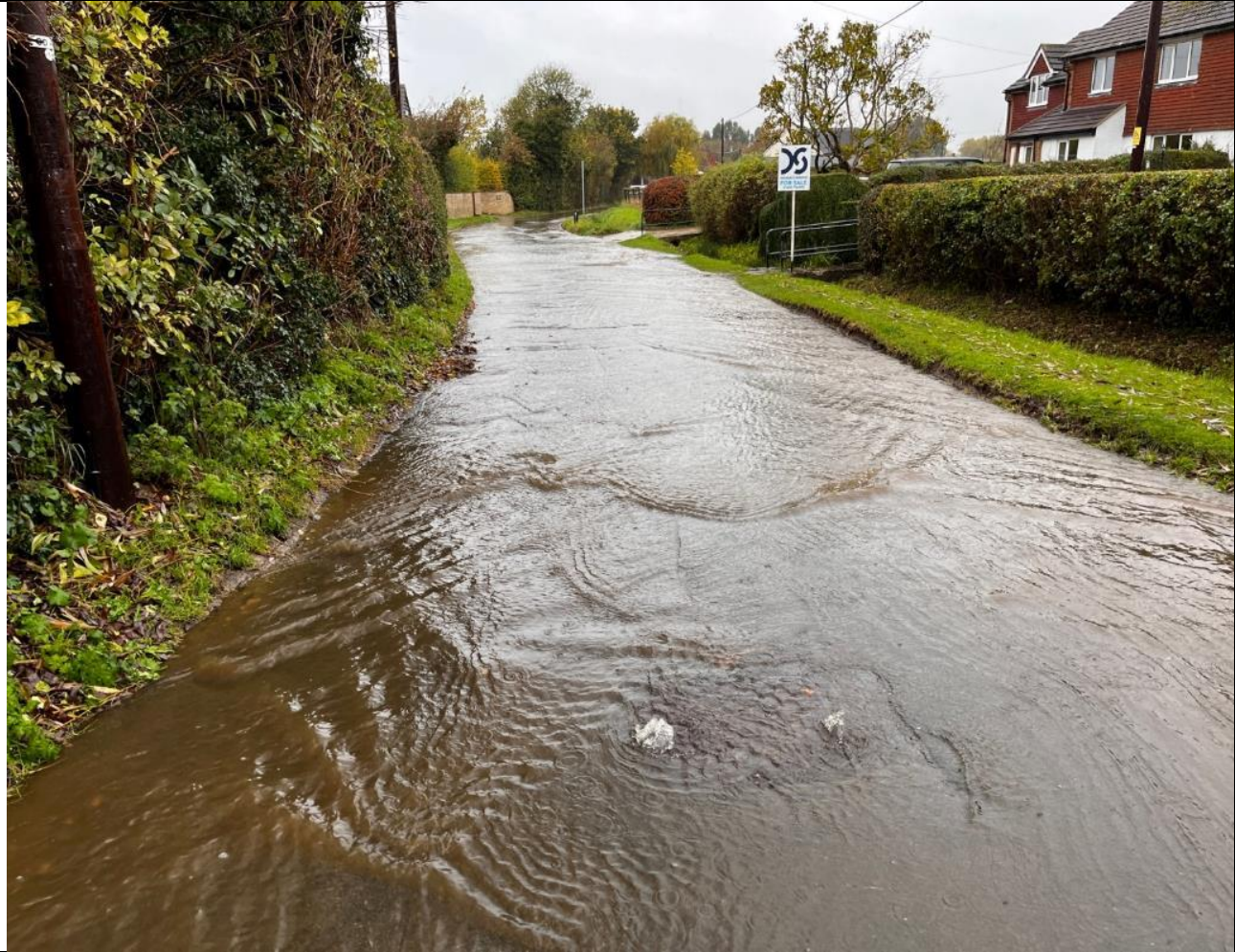
Woolstone Road/Shotover Corner – Nov 23 – note sewer bubbles from hydraulic flooding
