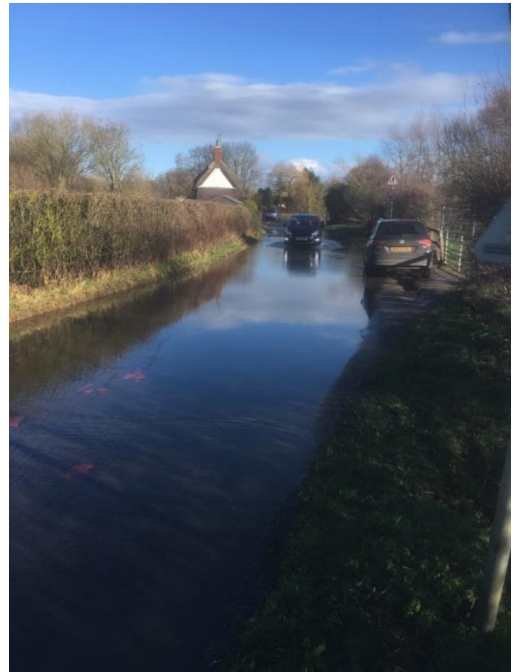
Woolstone Road outside Bridge Cottage – Jan 20
