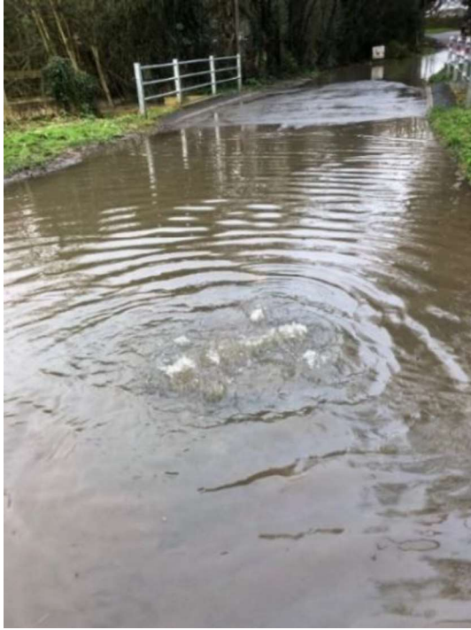
Flooding from the main sewer and damaged verge at allotments allowing the stream to overflow onto the Fernham Road – Feb 2024
