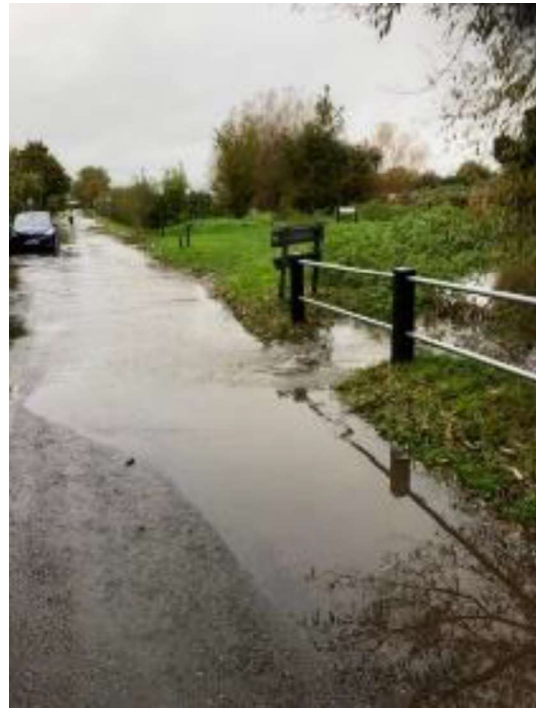
Flooding from the main sewer and damaged verge at allotments allowing the stream to overflow onto the Fernham Road – Feb 2024
