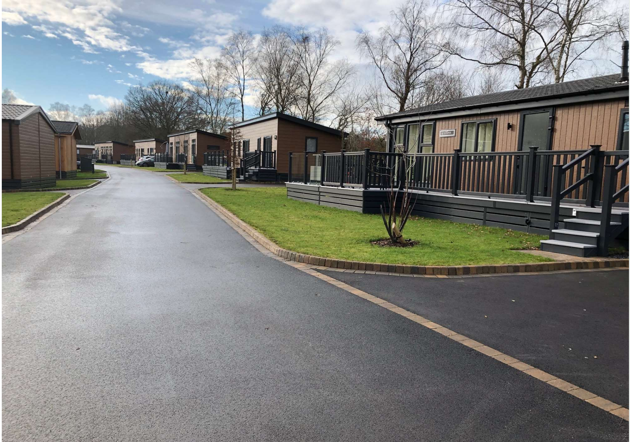
A typical Lovat Parks site
