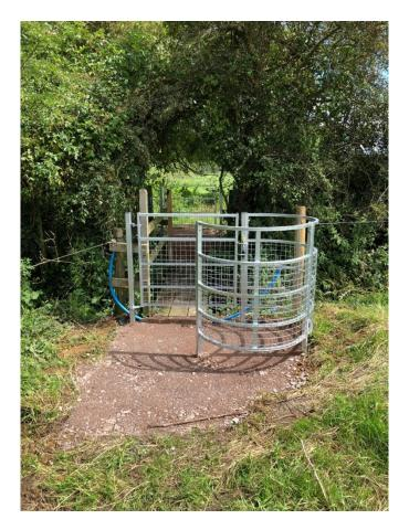
Note the blue hose, providing a safe conduit for the electrified wire, where required, under all the new gates.
