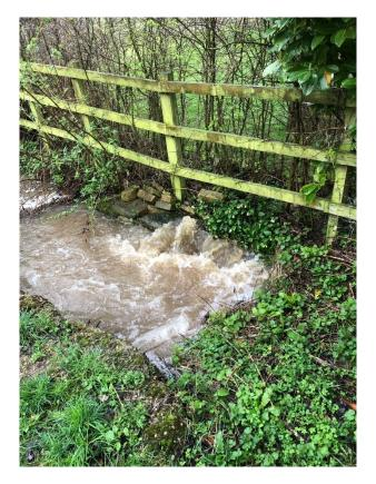
Photo 7. Entrance to the second culvert close to Stonehaven on 18 February 2024 – overloaded, and water unable to get away promptly.
