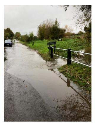
Photo 2. Damaged verge (at allotments) allows the stream to overflow onto the Fernham Road.
