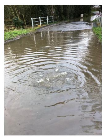
Photo 10. Hydraulic flooding from the main sewer, polluting the Uffington Brook outside Field House SN7 7RD on 18 February 2024.
